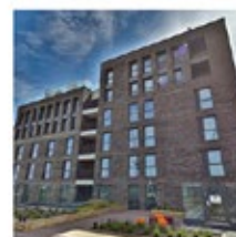
Berol Yard, Tottenham Hale. Value £38M View Project ▸
