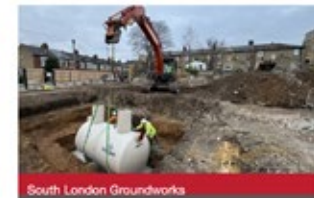
South London Groundworks
