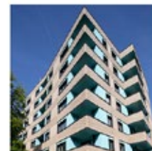
Hoylyn Square, Tower Hamlets. Value £11M View Project ▸
