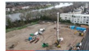
Kew Riverside CFA Bearing Piles | 350, 400 & 450mm | Depth up to 24.5m
