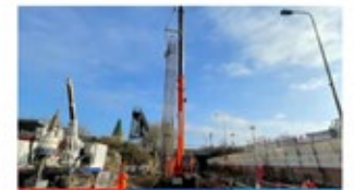
Botley Road Bridge
